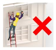
Figure 3 Incorrect – overreaching and not maintaining three points of contact
