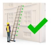
Figure 5 Check all sections are locked before using the ladder
